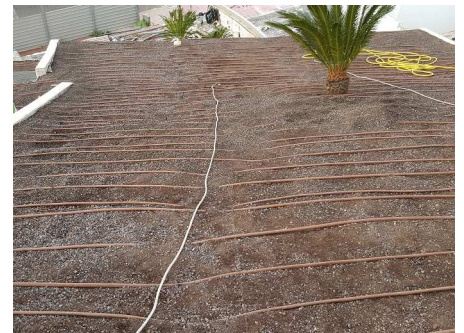
Two coordinated irrigation systems were installed for optimising the water supply.
