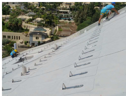
More than 700 Shearfix LF 300 support brackets had to be installed on the steep pitched roofs.
