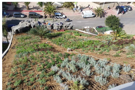
Detailed view of the shear barriers with TRP 80 eaves profile, Georaster and WSM 150 Mat.
