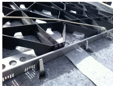
Detailed view of the shear barriers with TRP 80 eaves profile, Georaster and WSM 150 Mat.
