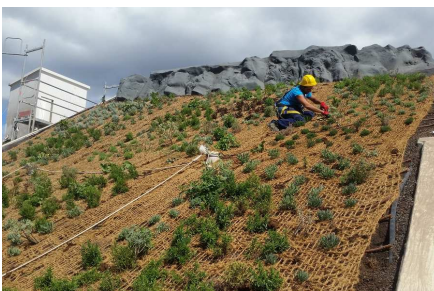
More than 700 Shearfix LF 300 support brackets had to be installed on the steep pitched roofs.
